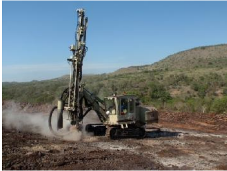
Drilling and blasting
